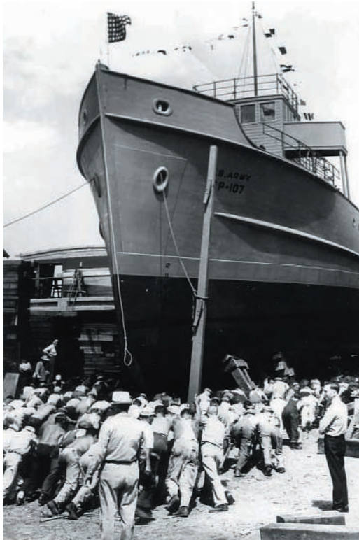
One of three 144' Army Troop/Cargo ships built at Minneford during World War II being readied for launching with aid of all hands in the yard. These were among the largest displacement vessels turned out at City Island.
